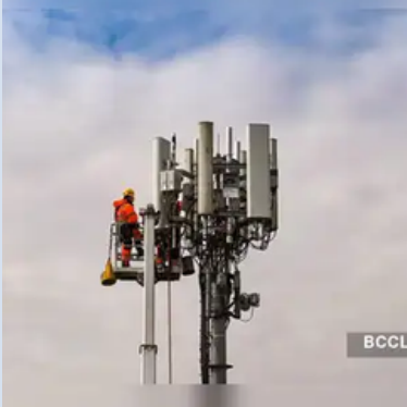
4TH SECTOR ADDITION
